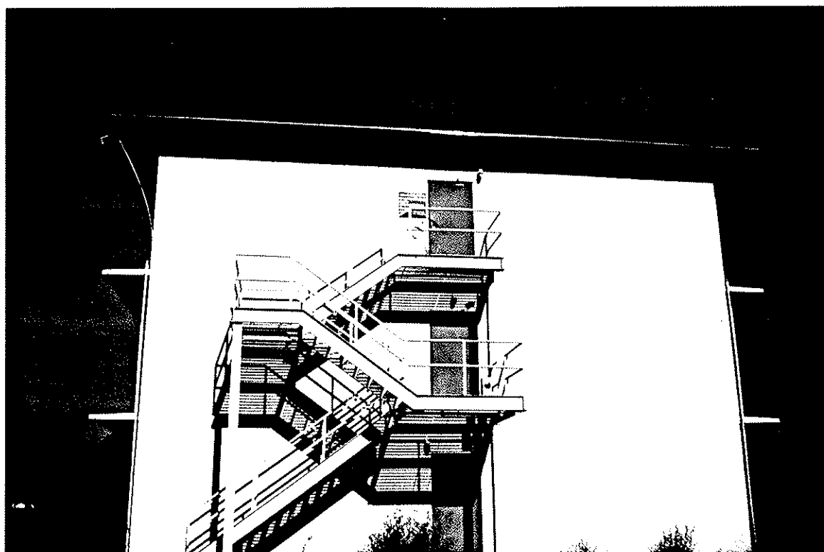
2. Facility 977, exterior side view.
