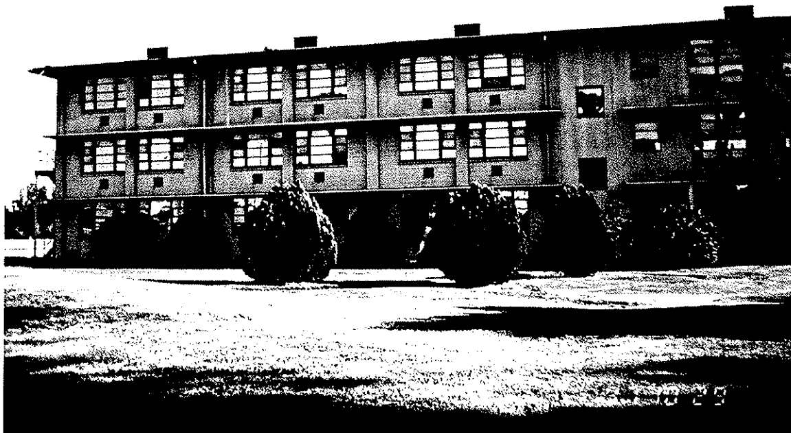
1. Facility 977, exterior front view.
