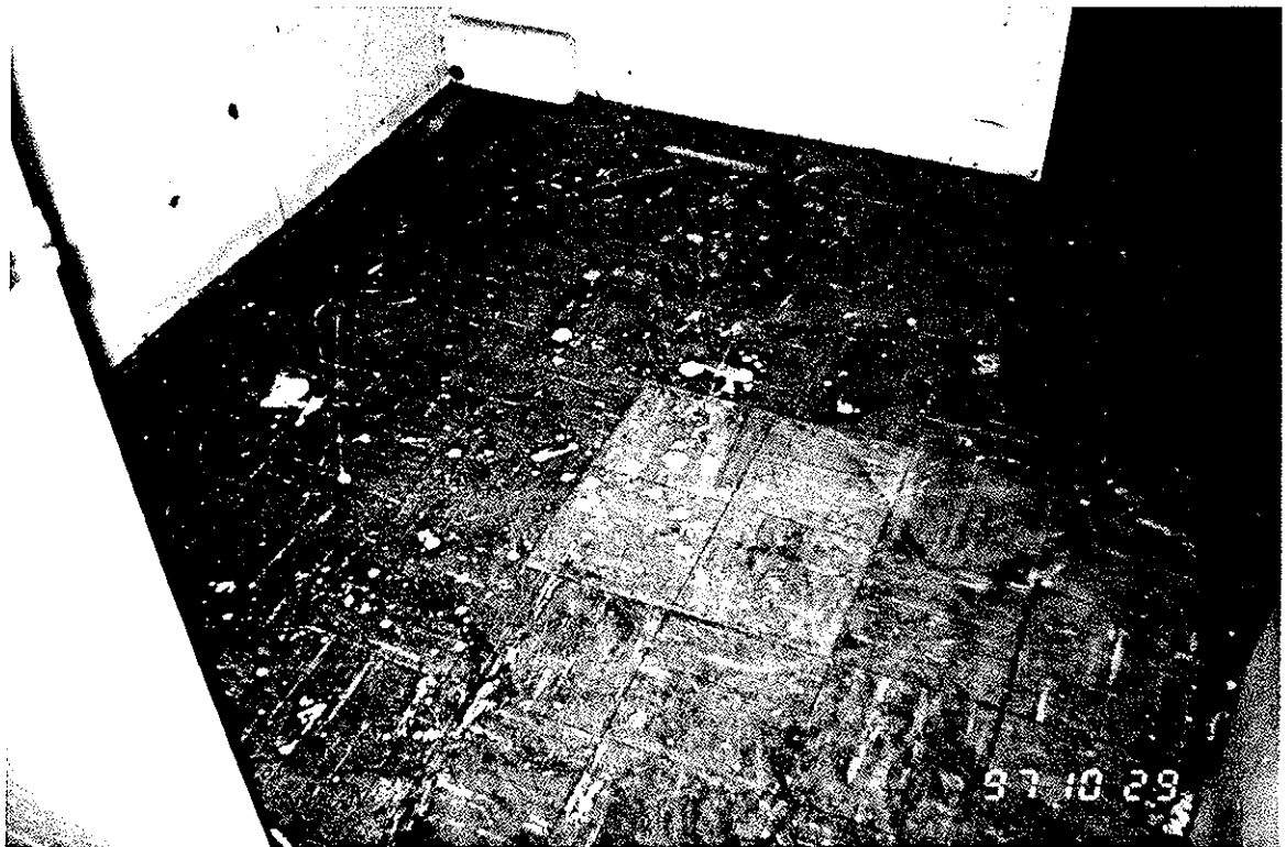
4. Facility 977, damaged 9" green VFT/mastic.
