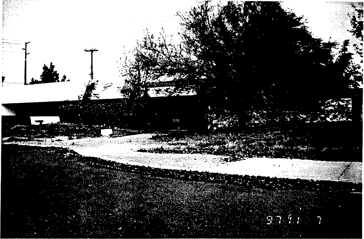
1. Facility 2995, exterior front view.
